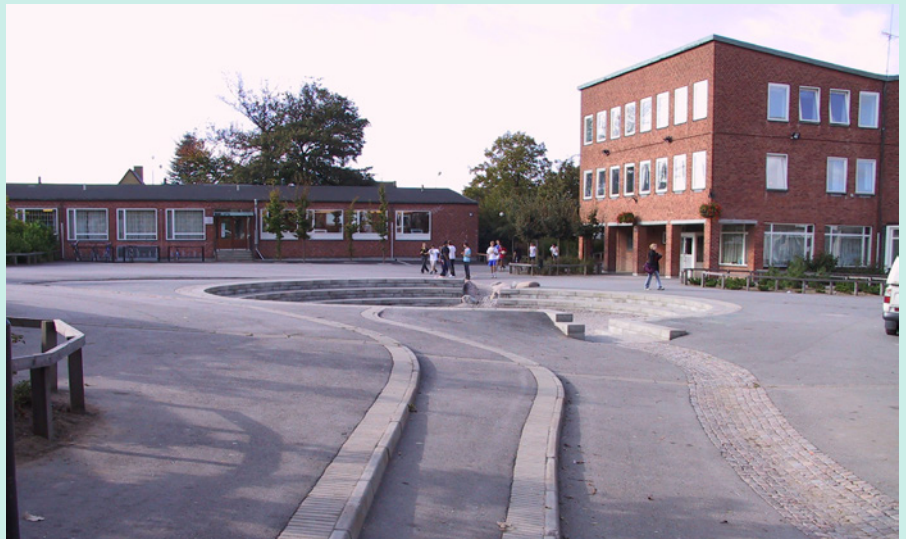
Stormwater reservoir constructed in an existing schoolyard, Augustenborg, Malmö. Credit: Tim Delshammar
